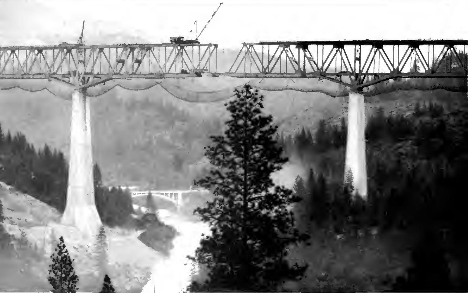
View of Pit River Bridge taken just as the central span was being placed connecting up the world's highest double deck structure
